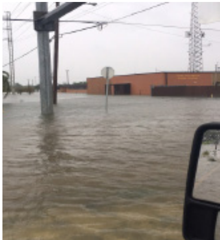
The TNMP office in Texas City was seriously damaged by flooding caused by Hurricane Harvey. TNMP crews worked tirelessly to restore power to impacted areas, despite the fact many were also dealing with personal challenges caused by the storm.
