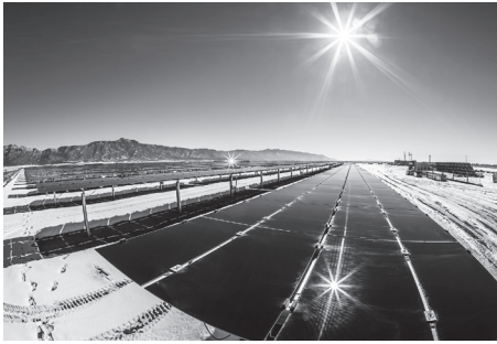
PNM's new solar generation facility at Meadowlake, NM uses state-of-the-art tracking technology to maximize electricity production.
