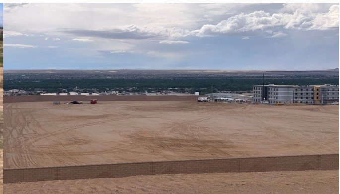
Site Ready for a Substation
